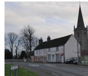
Figure 16 Grade II Listed 1 The Street (Church Cottage)
