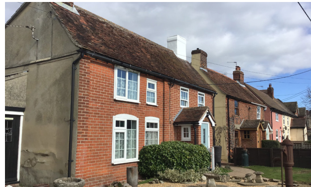
Figure 26 The nineteenth century cottages with a variety of red brick and painted render elevations with clay roof tiles
