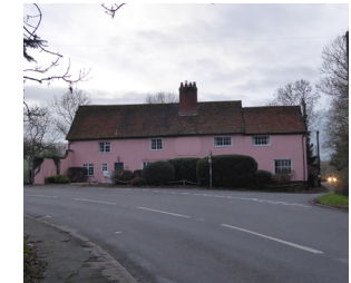
Figure 15 Grade II Listed Crown House
