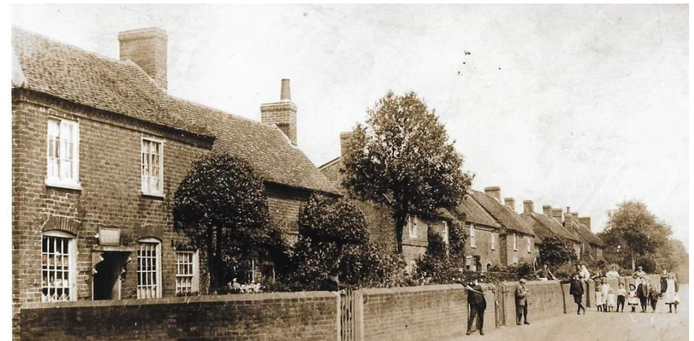
Figure 8 Row of nineteenth century cottages - early twentieth century- with the original red brick boundary wall. Grove Cottage, without the existing fake timber cladding, occupies a prominent position at the western end of the group.
